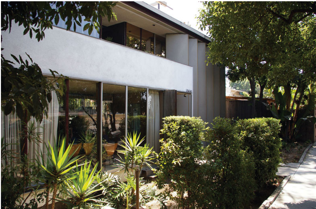
Fig. 15. Los Angeles, Richard Neutra's VDL Research House II, showing vertical sun-shading devices at far right (author's photograph, 2009)
